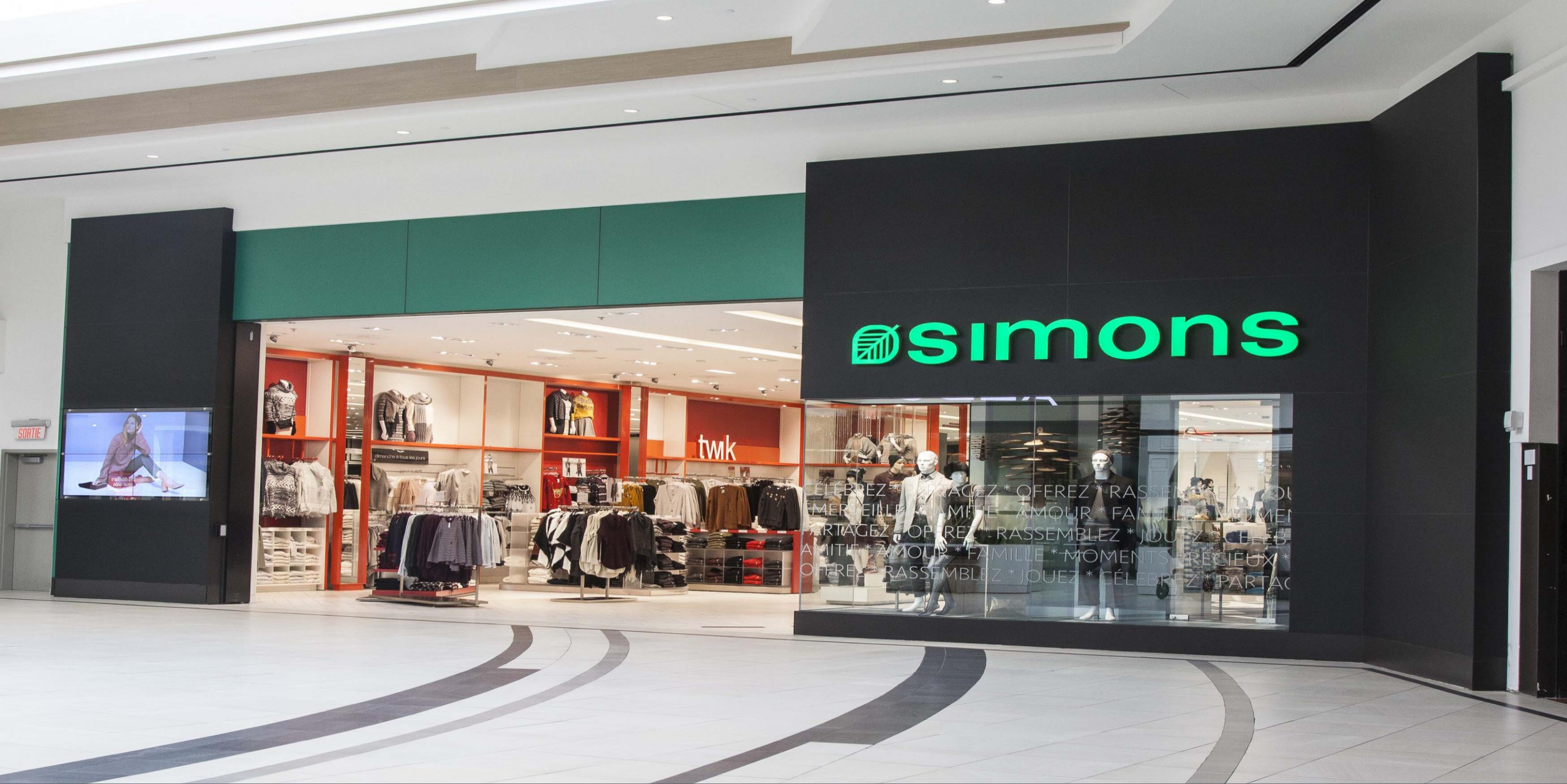
Simons Store – Gatineau, QC 6mm low-iron acid-etched glass, back painted and tempered
