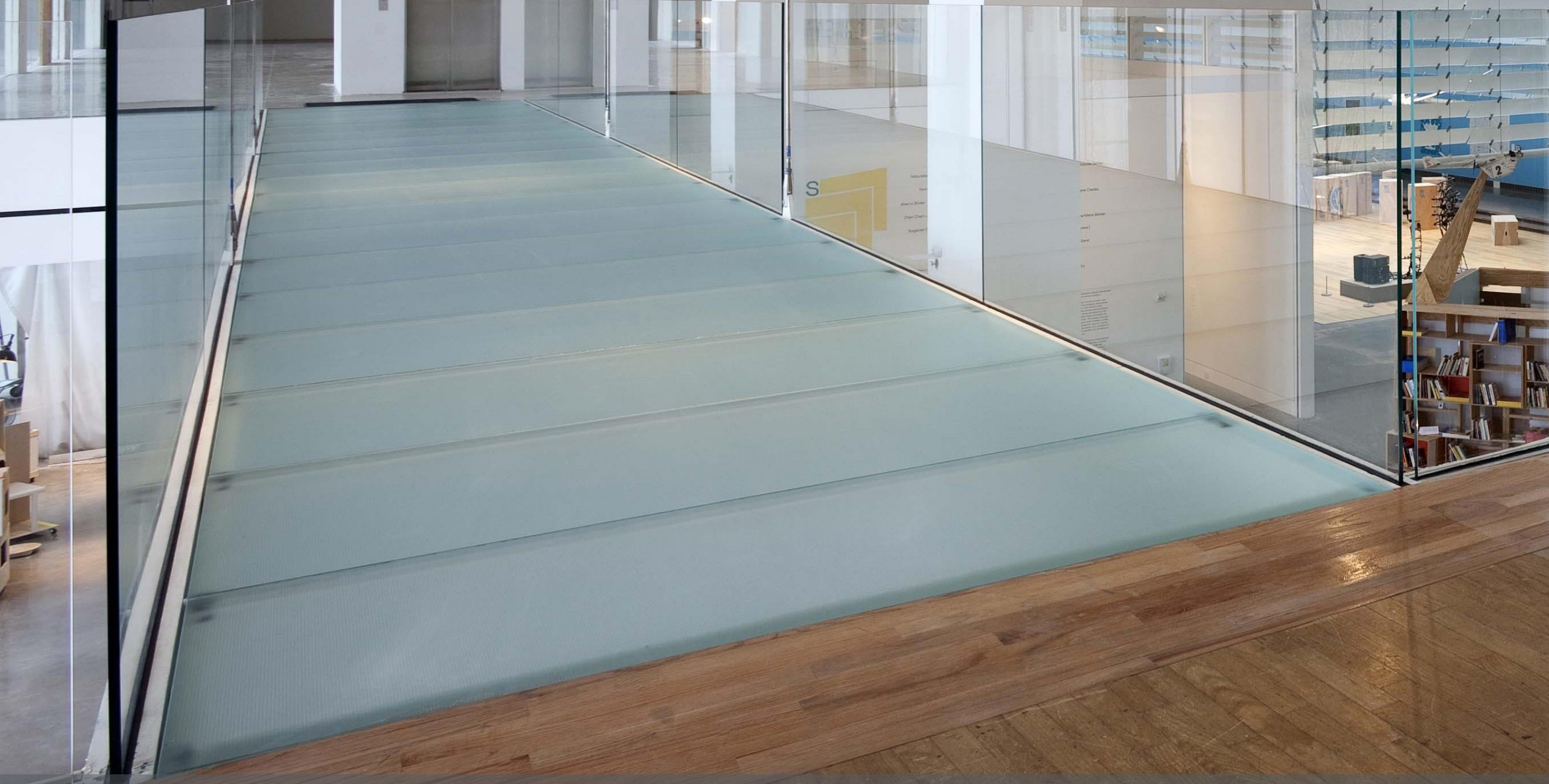
Queens Museum – Queens, NY 12mm Starphire glass with pattern 406, tempered and laminated
