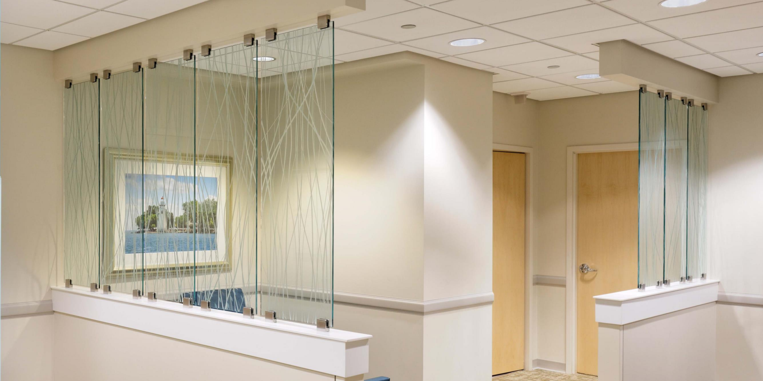
Firelands Regional Medical Center – Sandusky, OH 12mm clear glass with acid-etched pattern 512, 2 faces
