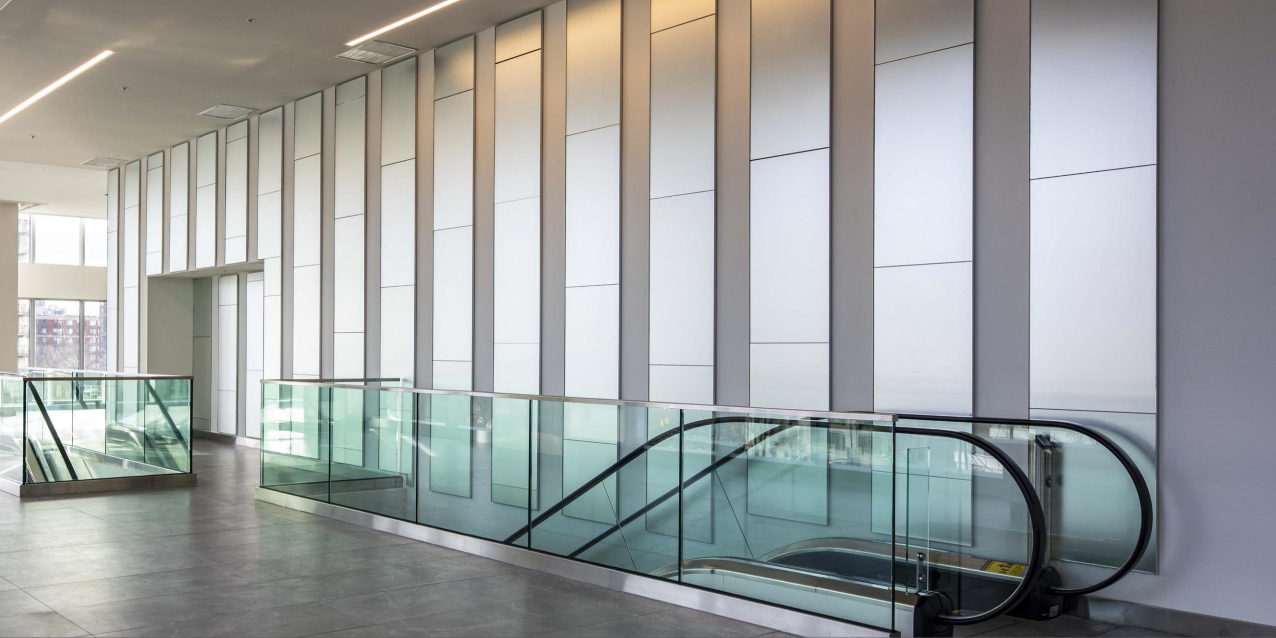
TDC2– Montreal, QC 6mm low-iron mirror with acid-etched Satin finish
