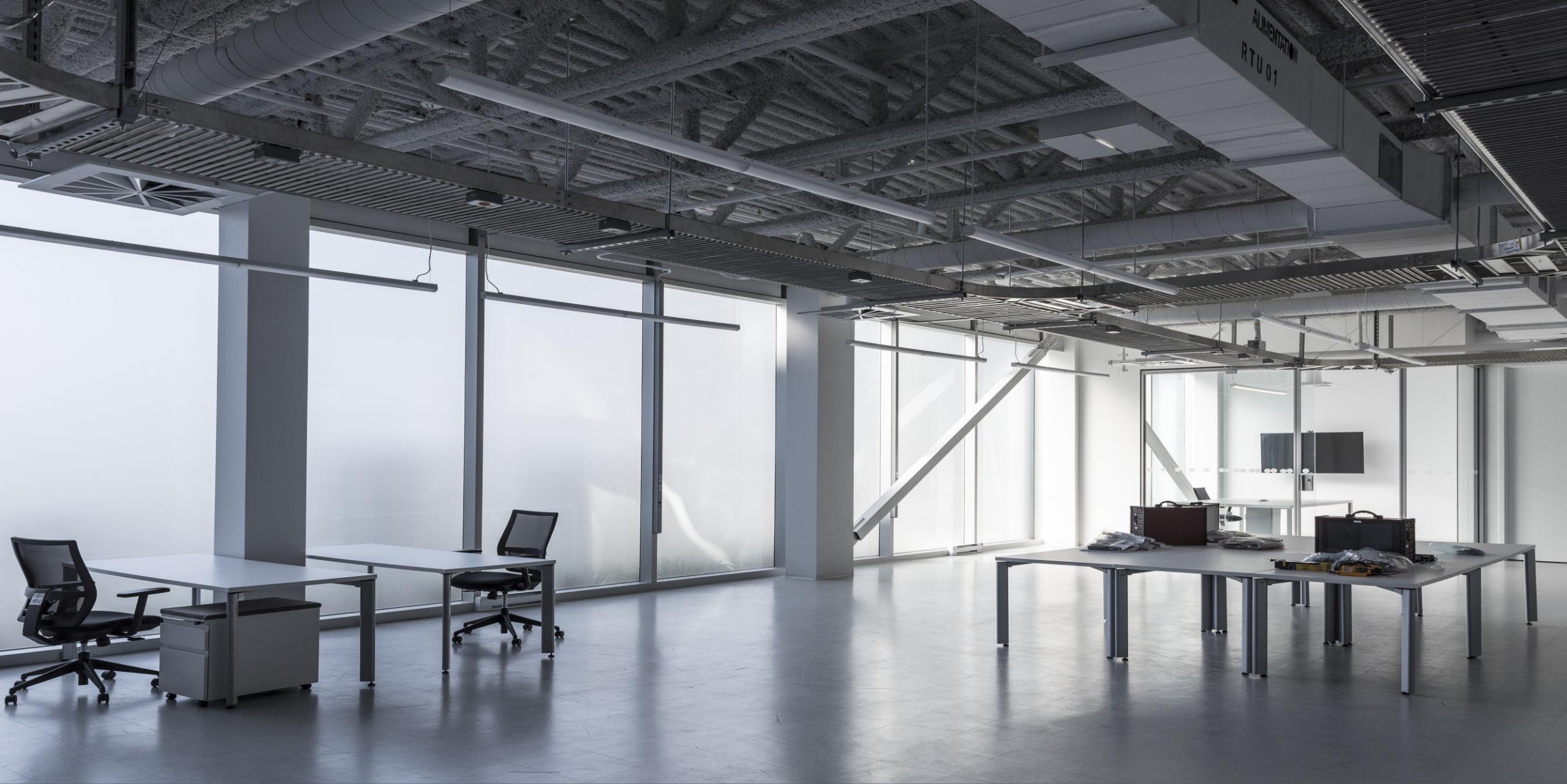
ABB Canada Campus – Montreal, QC Insulated Glass Unit – 6mm Starphire Ultra-Clear™ Opaque Surface #2
