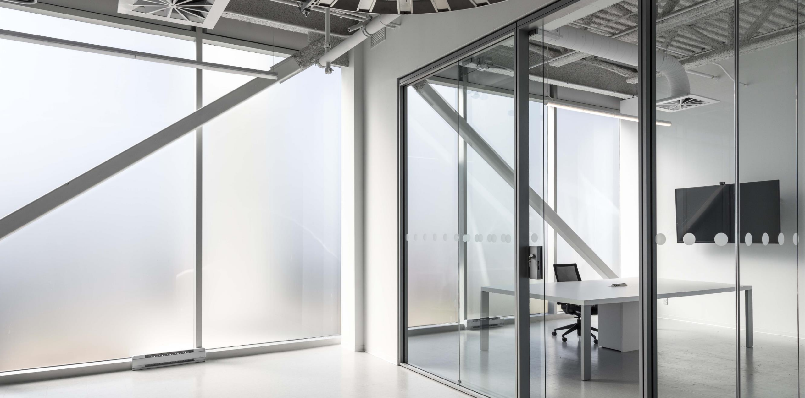
ABB Canada Campus (LEED® Gold Certified) – Montreal, QC 6mm Starphire Ultra-Clear™ glass Opaque finish on surface 2
