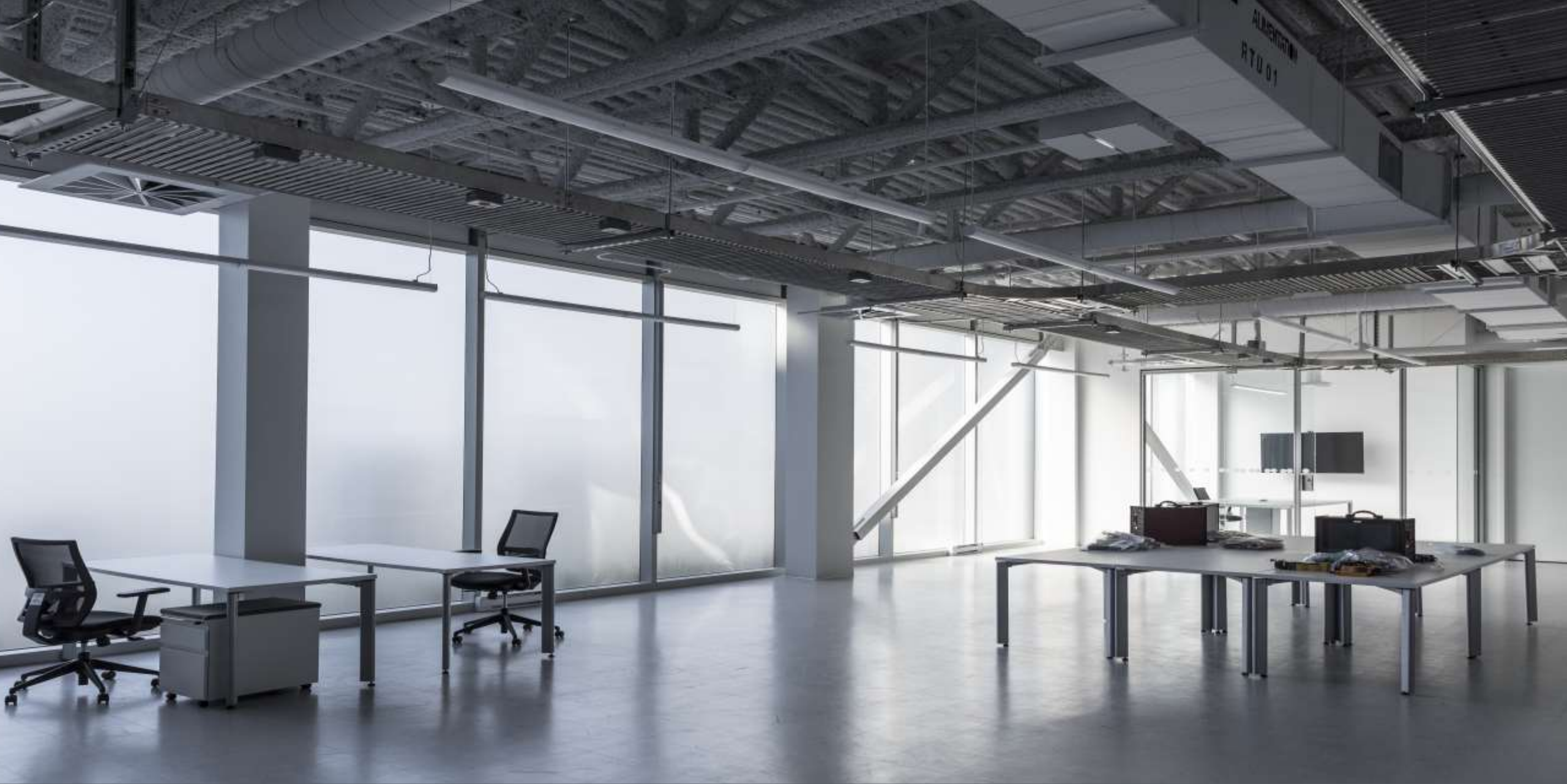
ABB Canada Campus – Montreal, QC Insulated Glass Unit – 6mm Starphire Ultra-Clear™ Opaque Surface #2
