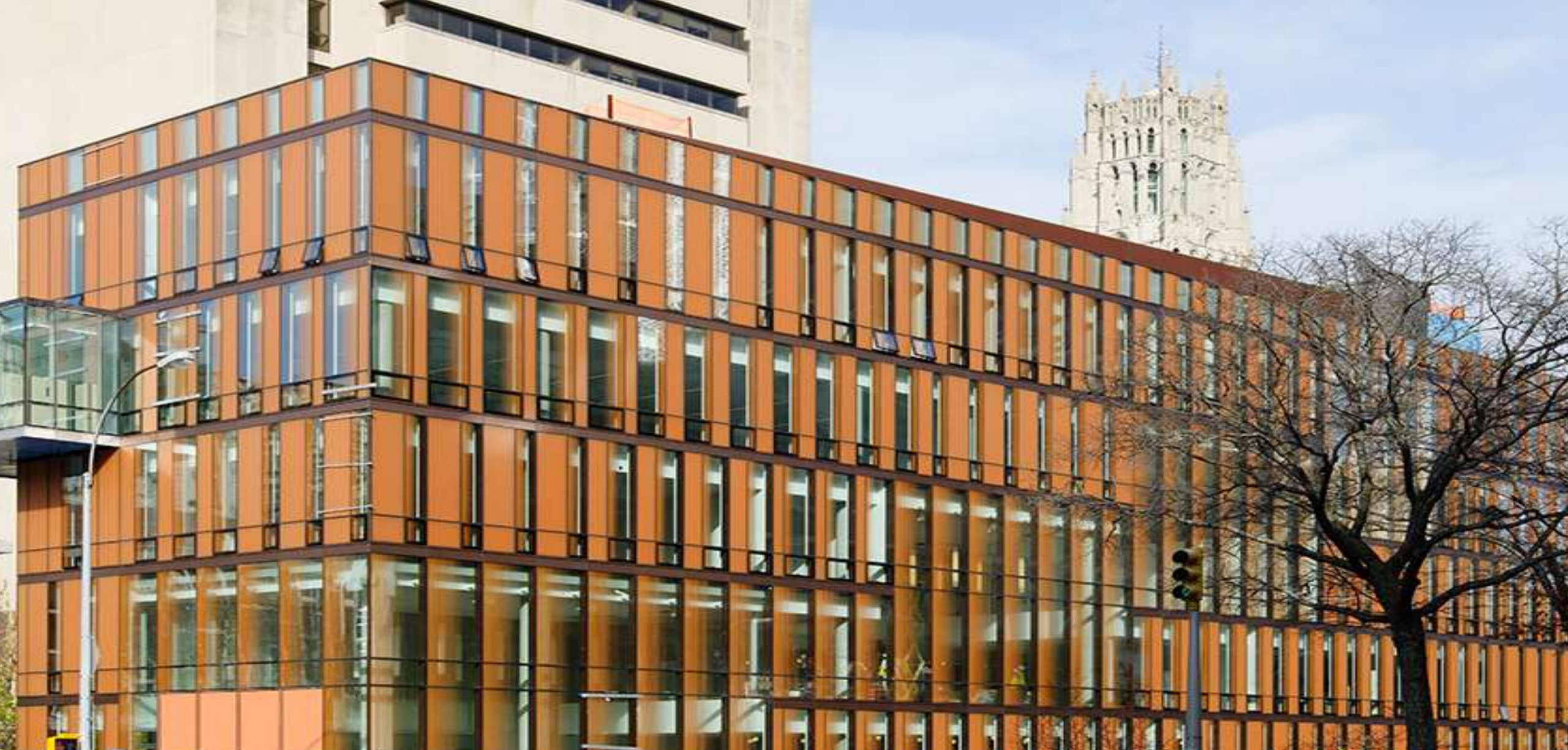
Diana Center Barnard College – New York, NY Insulated Glass Unit – 6mm Starphire Ultra-Clear™ Glass Velour Surface #1, Terracotta Ceramic Paint Surface #2, Tempered , Solarban® 60 Surface #3
