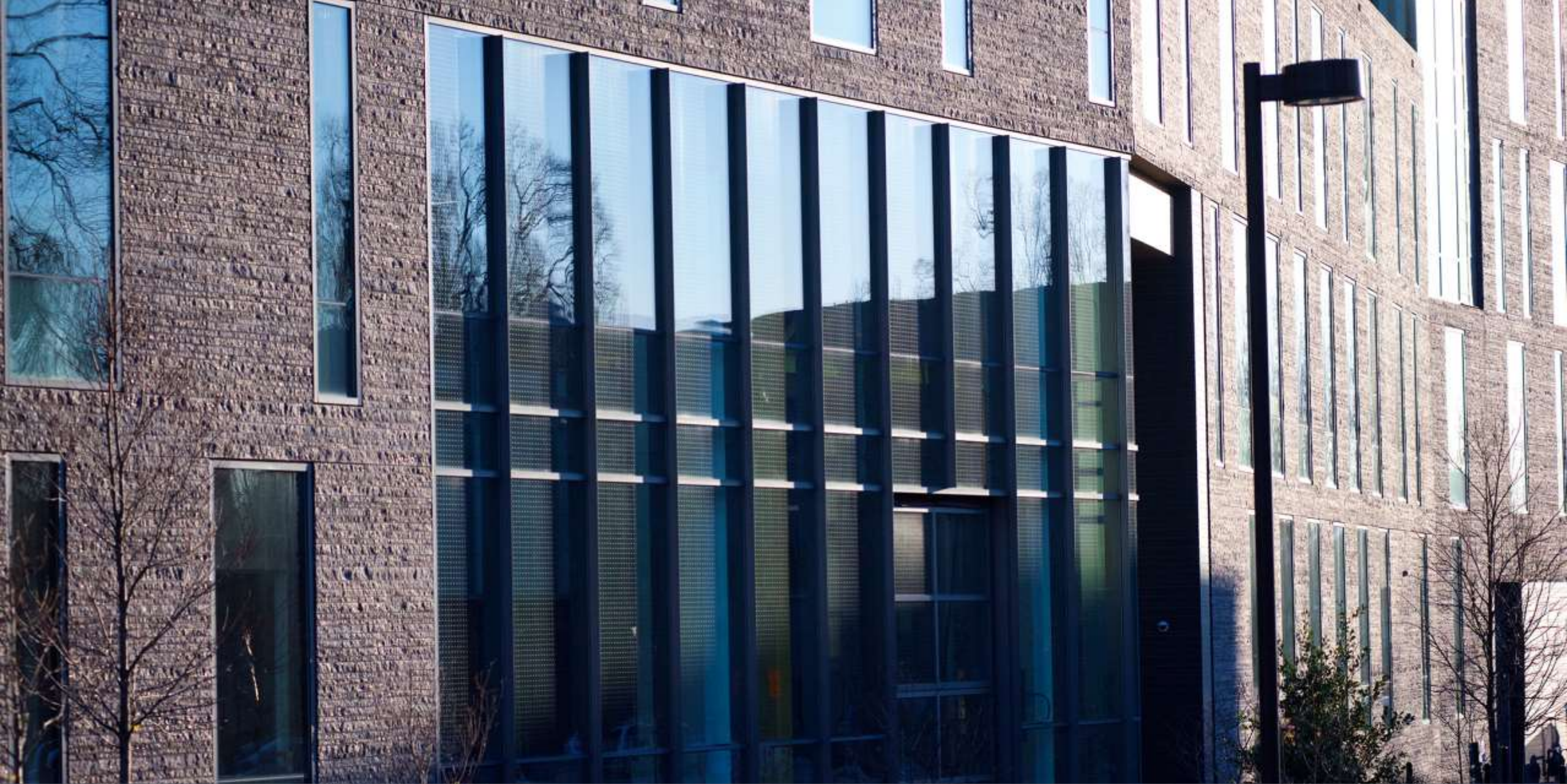
Swarthmore College Maxine Signer Hall – Swarthmore, PA Insulated Glass Unit – 6mm Clear Glass AviProtek® E pattern 215, Solarban® 60 on surface 2
