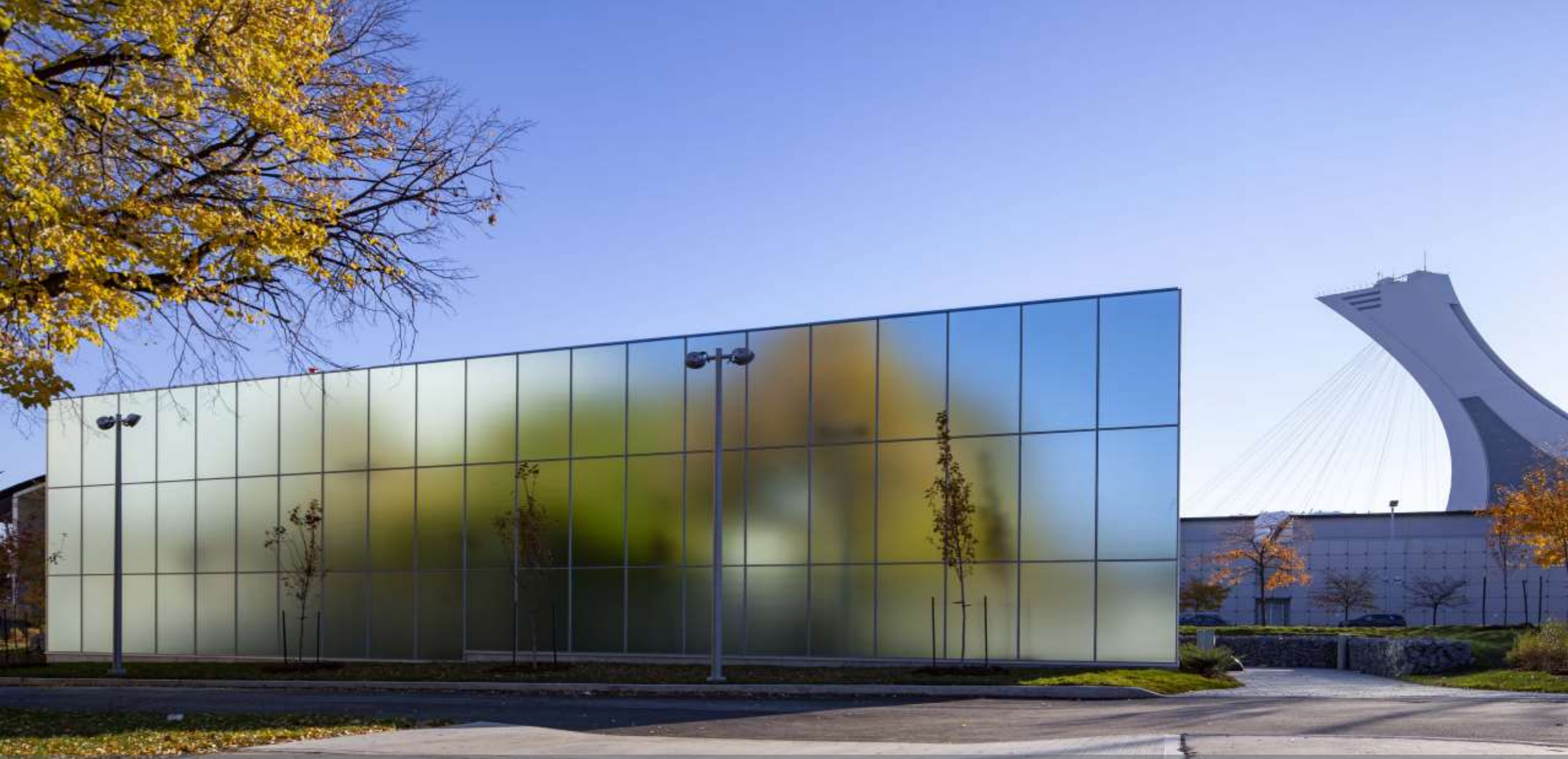
Maurice Richard Arena – Montreal, QC 6mm clear glass Satinlite on surface 1 with 6mm grey glass Pilkington Mirropane™ on surface 3 backpainted in grey on surface 4
