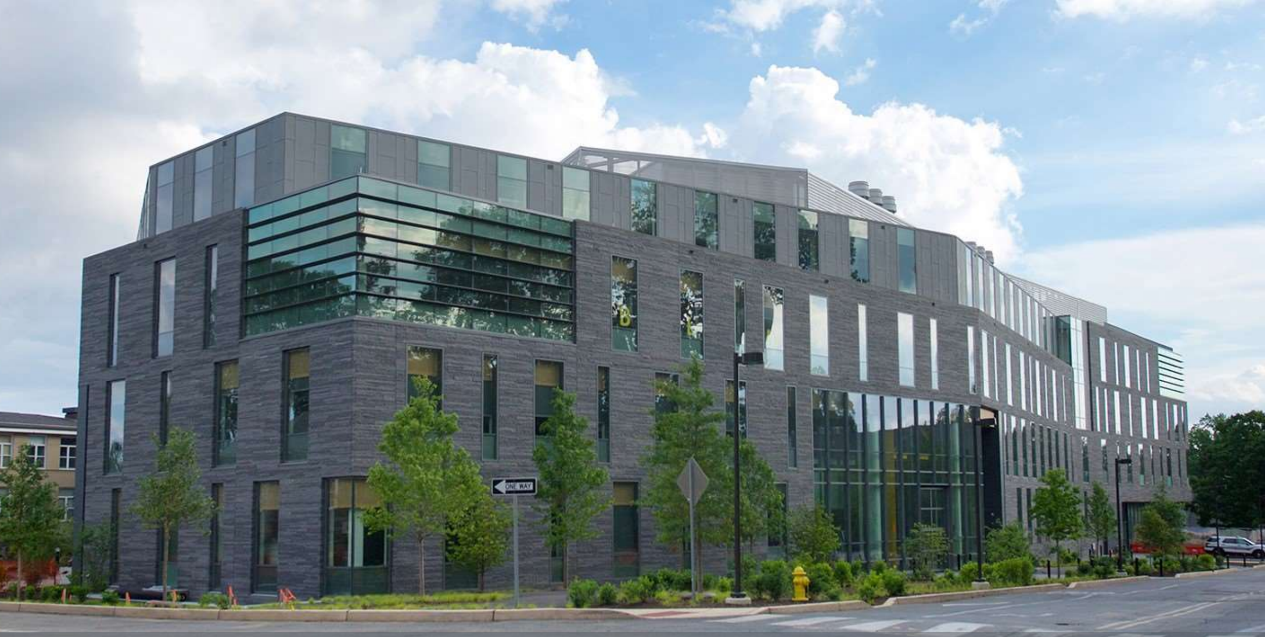
Swarthmore College Maxine Signer Hall – Swarthmore, PA Insulated Glass Unit – 6mm Clear Glass AviProtek® E pattern 215, Solarban® 60 on surface 2
