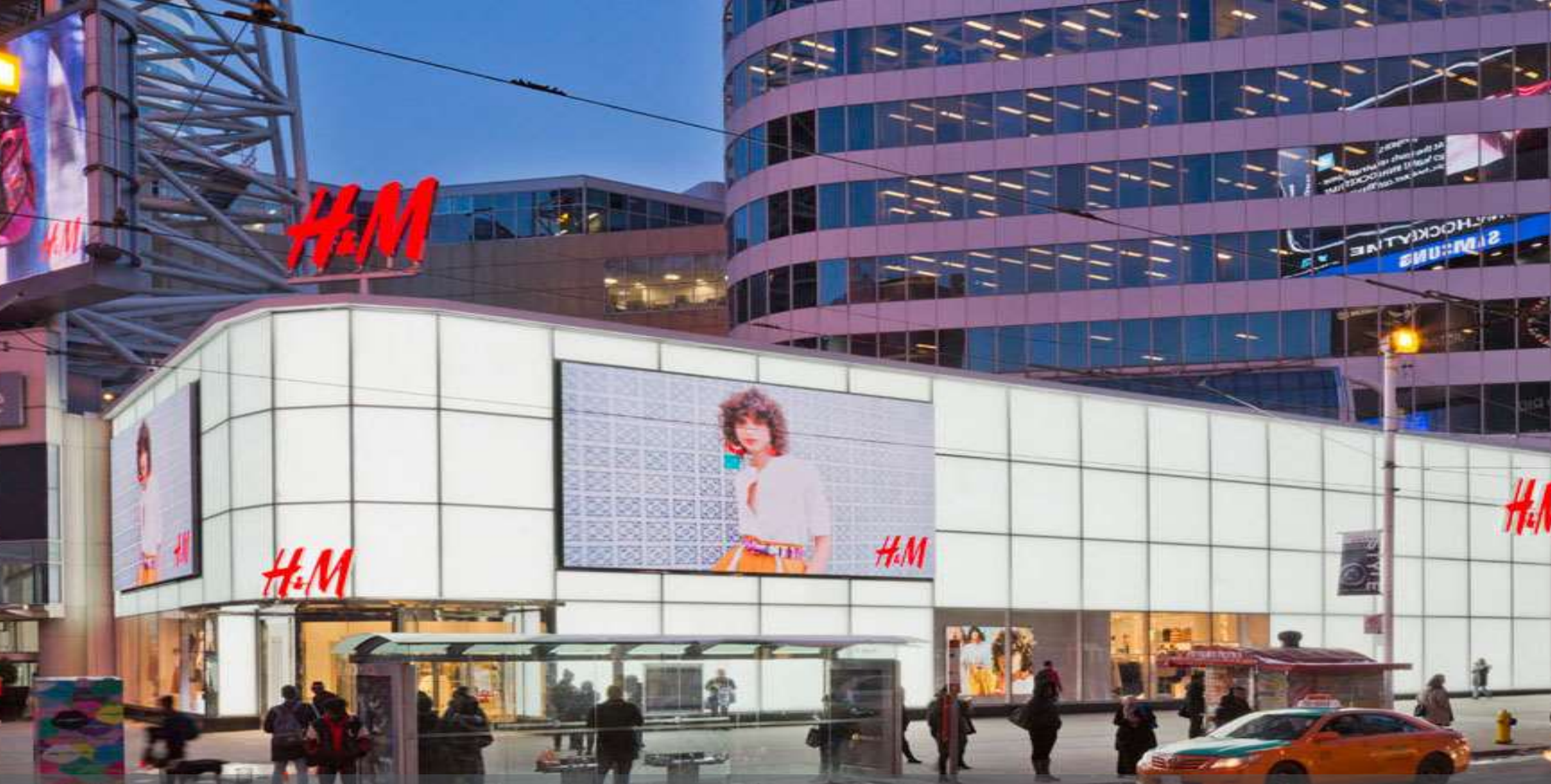
H & M Store – Toronto, ON Insulated Glass Unit – 8mm Starphire Ultra-Clear™ Opaque Surface #1, 2, 3 & 4
