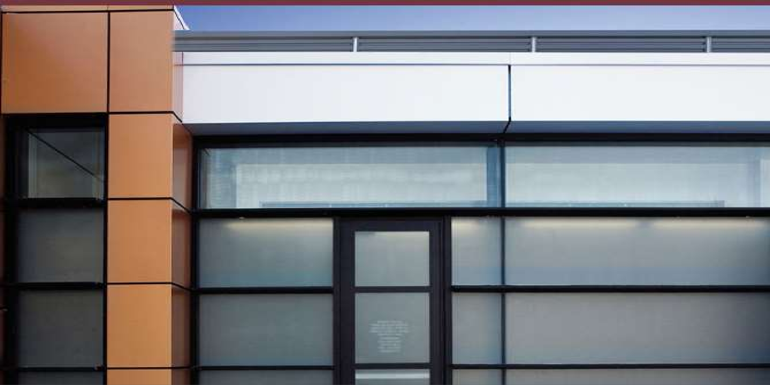
National Institute of Scientific Research (INRS) - Laval, QC Insulated Glass Unit – 6mm Starphire Ultra-Clear™ Satin Surface #1, Solarban® 60 Surface #3
