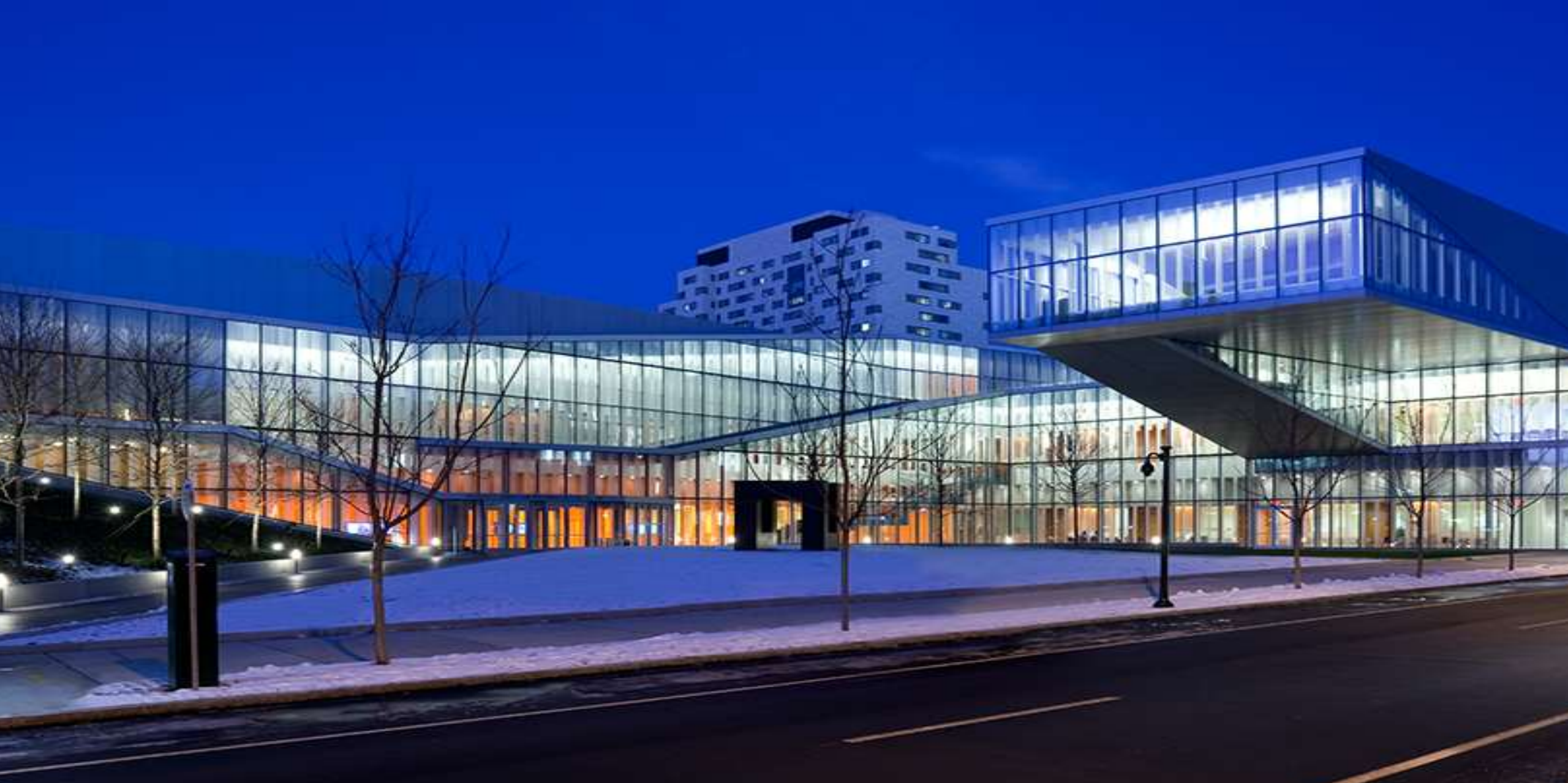
University of Pennsylvania – Philadelphia, PA Insulated Glass Unit – 6mm Starphire Ultra-Clear™ Nuance Custom Velour Stripes Surface #1
