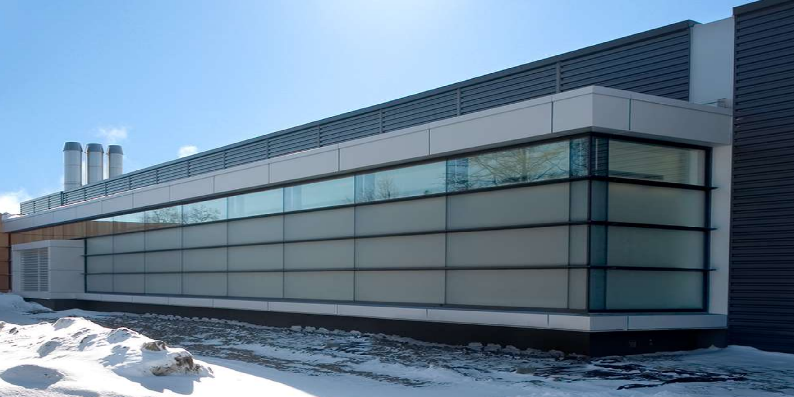
National Institute of Scientific Research (INRS) - Laval, QC Insulated Glass Unit – 6mm Starphire Ultra-Clear™ Satin Surface #1, Solarban® 60 Surface #3
