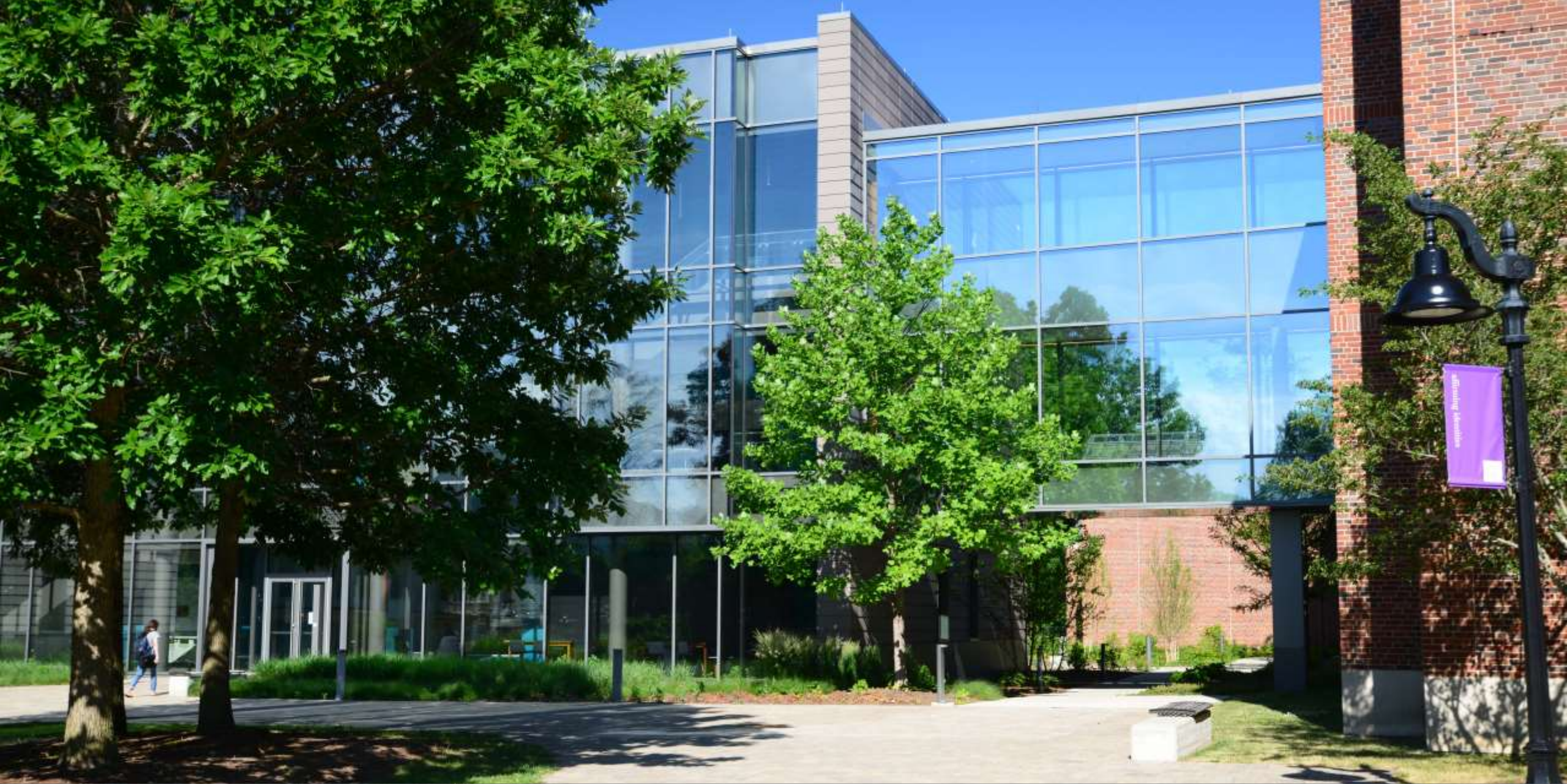
Williams College – Williamstown, MA Insulated Glass Unit – 6mm Clear Glass AviProtek® T pattern 713 on surface 1
