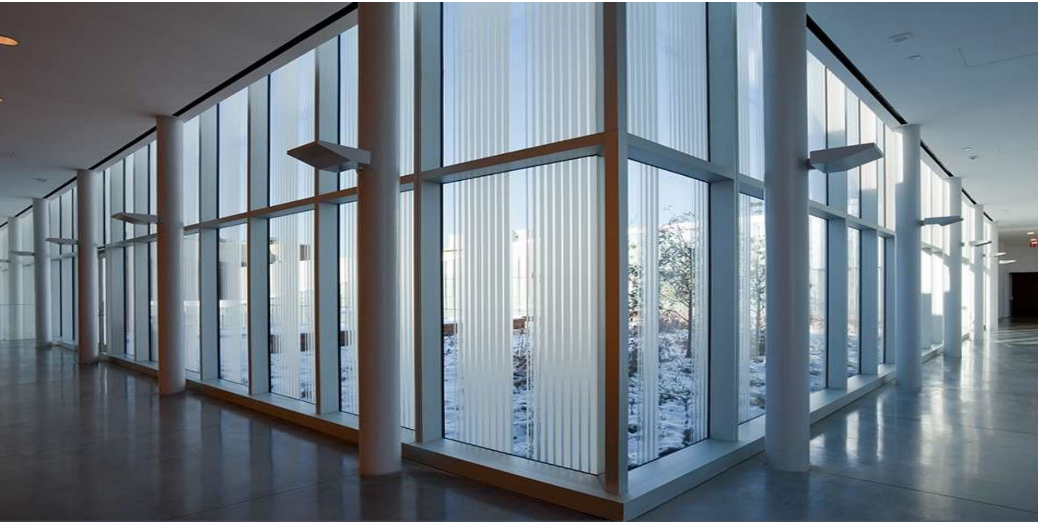
University of Pennsylvania – Philadelphia, PA IGU – 6mm low-iron glass with acid-etched stripes on surface 1
