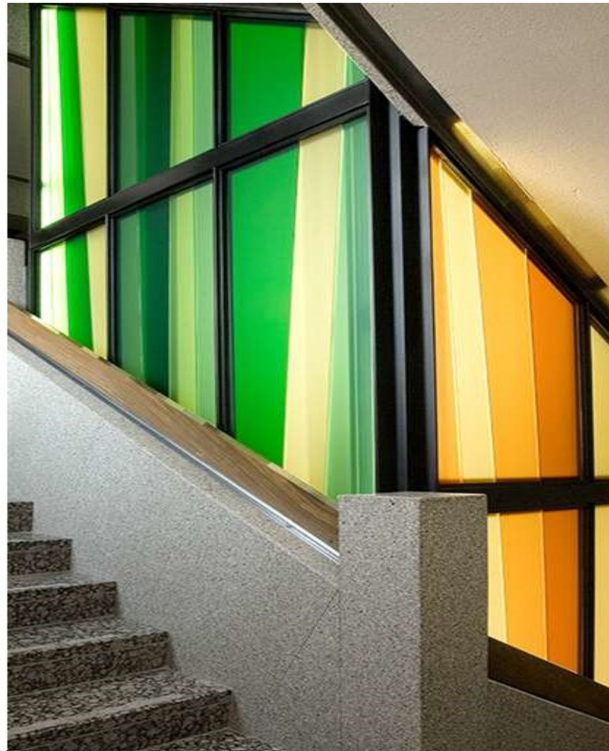
Saint Joseph's Oratory – Montreal, QC 6mm low-iron acid-etched glass, tempered & laminated with colored interlayers
