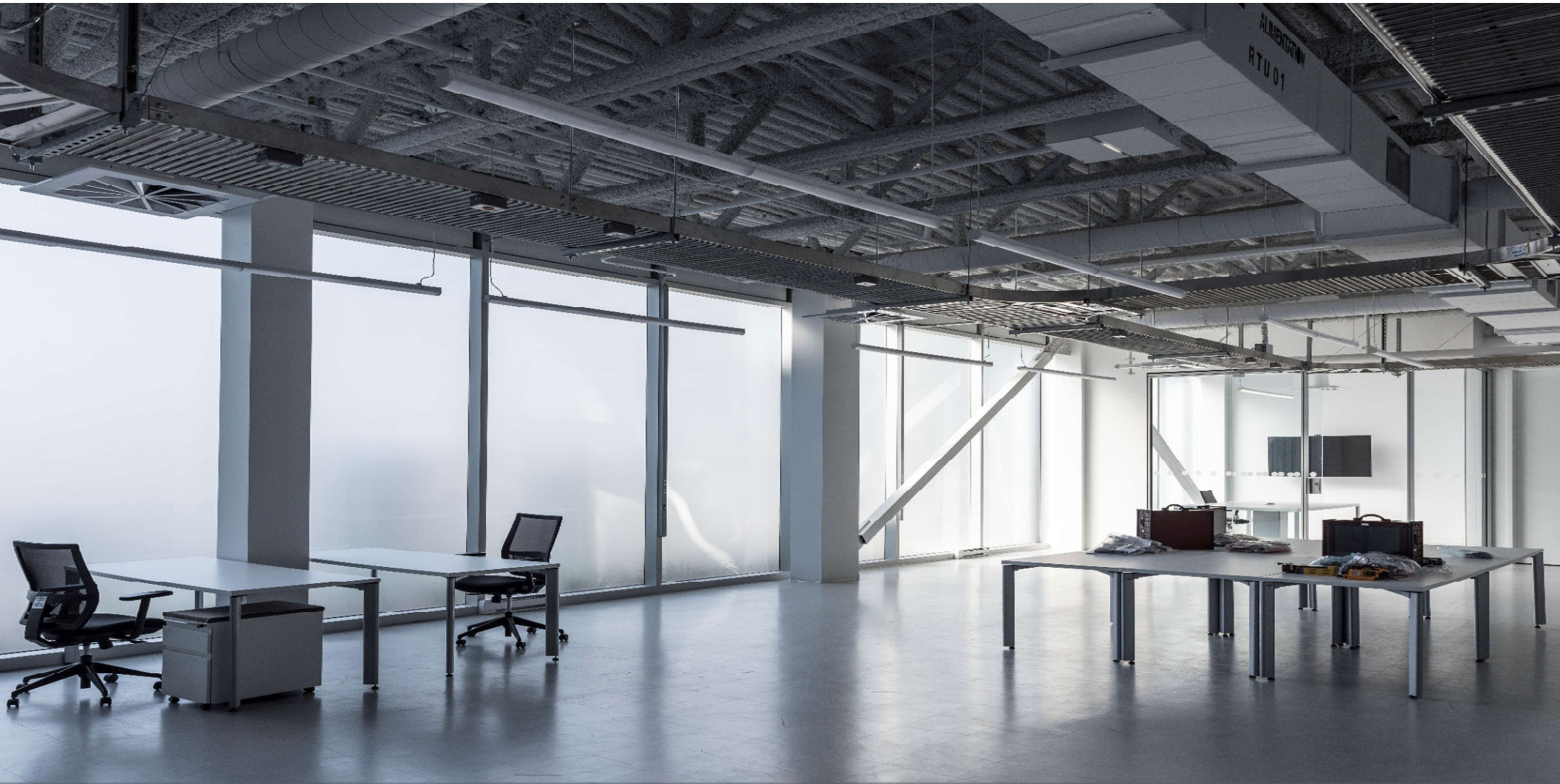
ABB Canada Campus – Montreal, QC IGU – 6mm low-iron acid-etched glass on surface 2, low-e on surface 3
