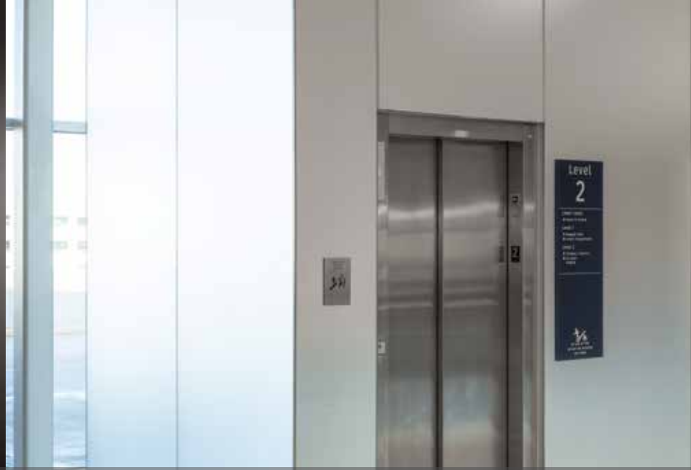
Will Rogers World Airport, Oklahoma, OK 6mm Starphire Ultra-Clear® mirror with Satin acid-etched finish
